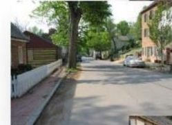
Lower pavement, fix drainage, protect trees
