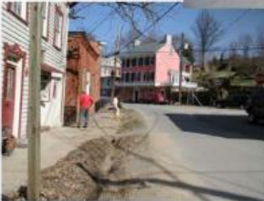
Lower pavement, fix drainage
