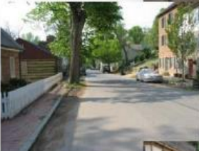
Lower pavement, fix drainage, protect trees
