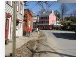
Lower pavement, fix drainage
